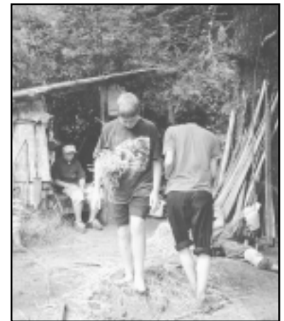
Keep on stomping! Mixing the straw and mud together to make cob.
