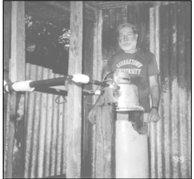
Ben and the completed Pelton wheel installation
